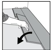
[6] Second plank, second row. Place the board tight to the short end of the previous panel. Insert the long end (tongue) into the first rows long end (groove). Insert at an angle then fold down in a single action movement
